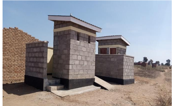
Improved pit latrines constructed at Kanjochi Primary School (left) and Mtsapira Market (right)
