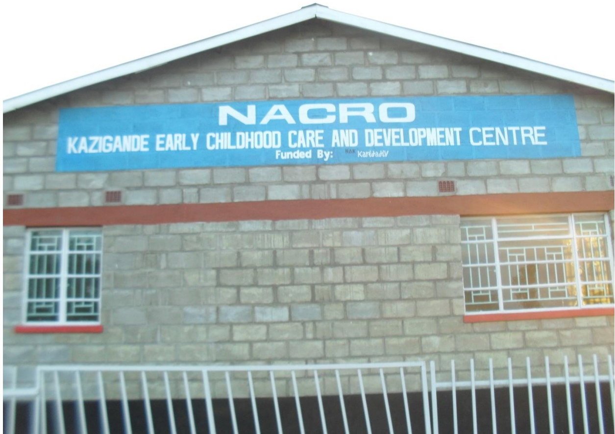
The classroom block
